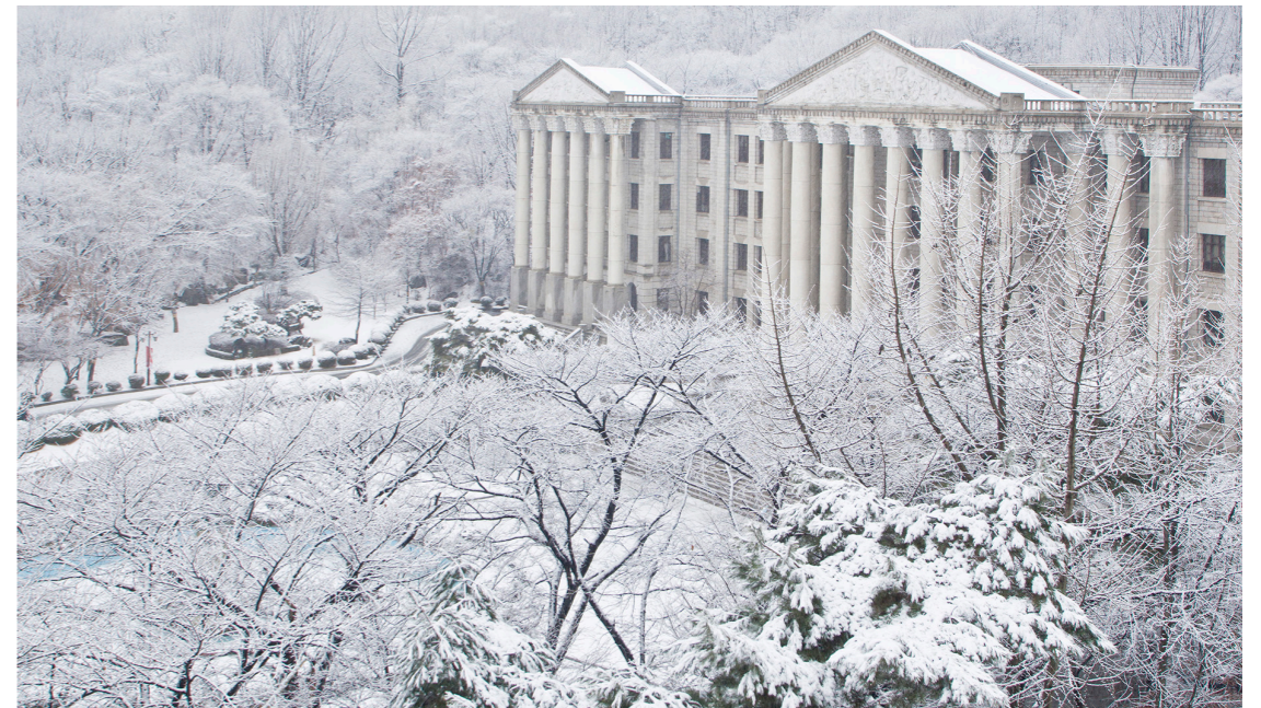
| Winter University Administration Building
